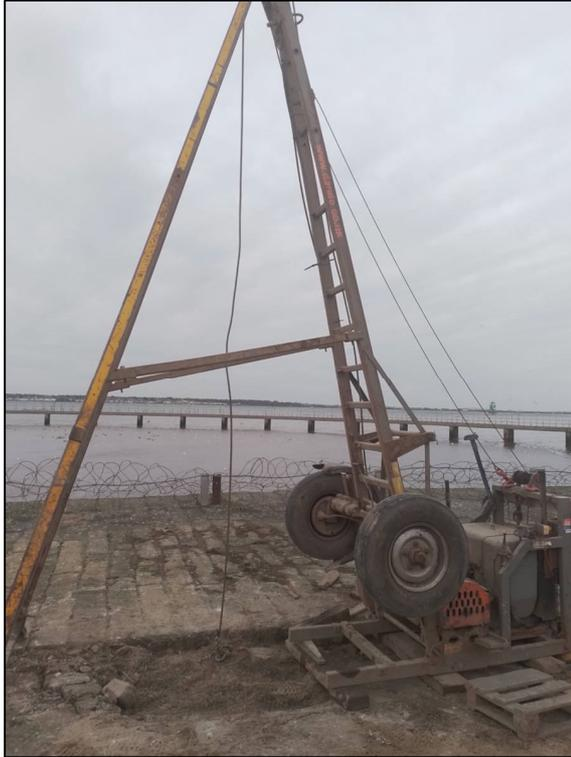
**Plate 11:** Cable percussion rig setup at BH-212 (Trench 7) on the landward side of GSW.
